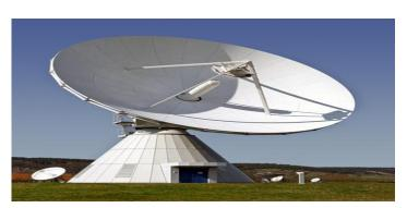
Radio telescopes are helping to provide data about the movement of the tectonic plates. The two stations are located on separate plates so the relative plate motion can be determined.
