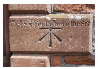
Bench Marks: These are marks placed on buildings, or on other places, indicating the height above sea level, determined by actual surveys. All the heights are determined by the surveys, ground surveys which are conducted by certain techniques recent techniques like total stations, theodolite and automatic level or GPS. On maps these are indicated by the letters B. M. followed by the height in feet or meters above
